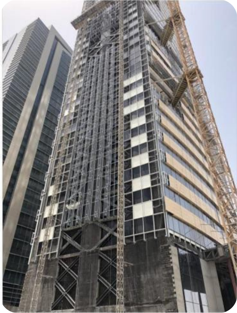
Building under construction photo
